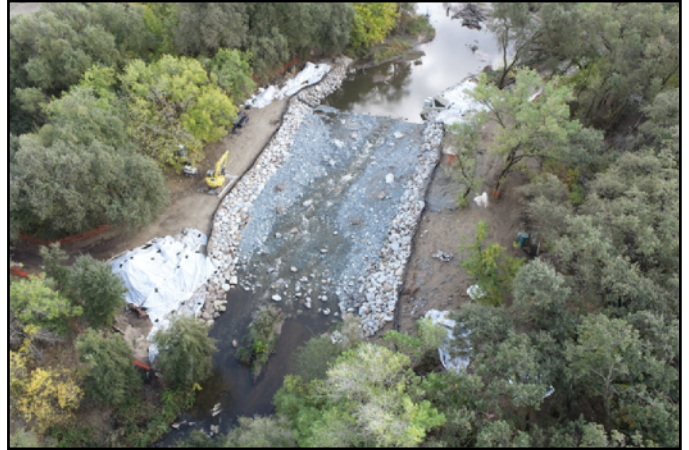
Hemphill Dam after rehabilitation. Image courtesy ECORP Consulting, Inc.
